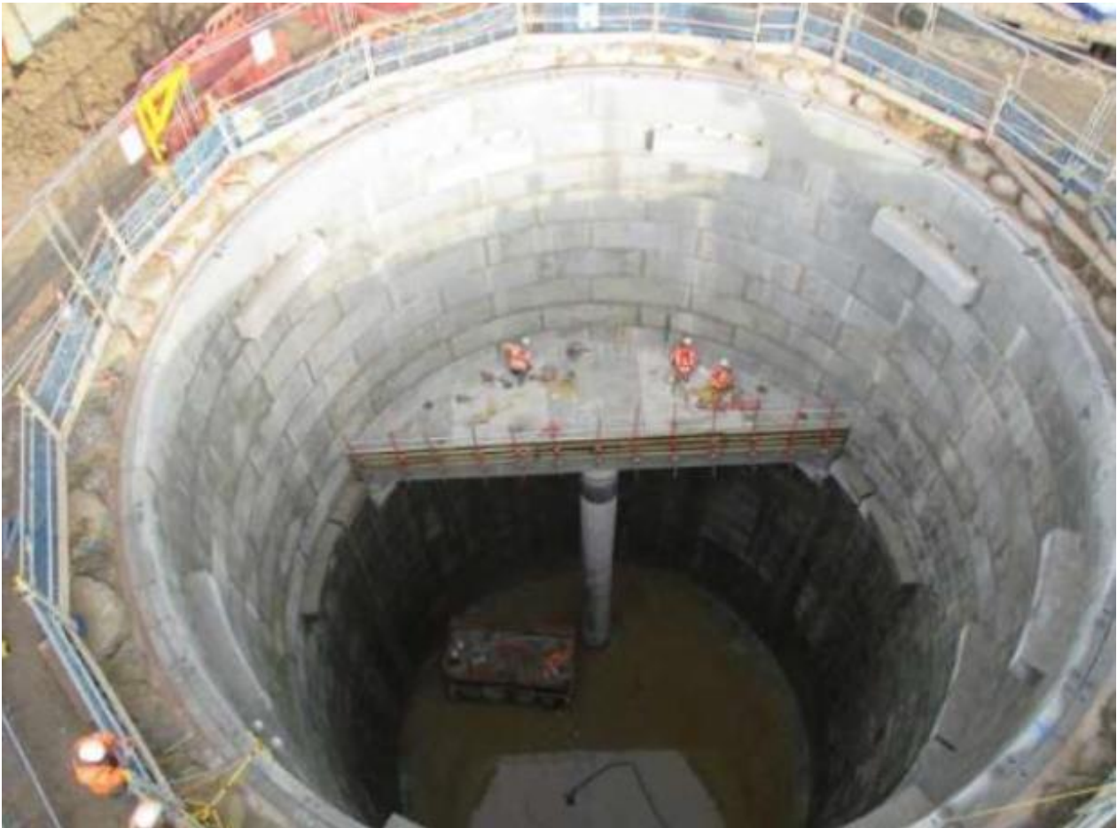
Figure 18 - Underground storage tank under construction
