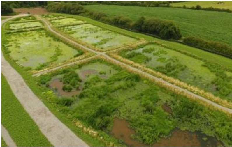
Figure 54 - Cromhall WRC – Integrated Constructed Wetlands
