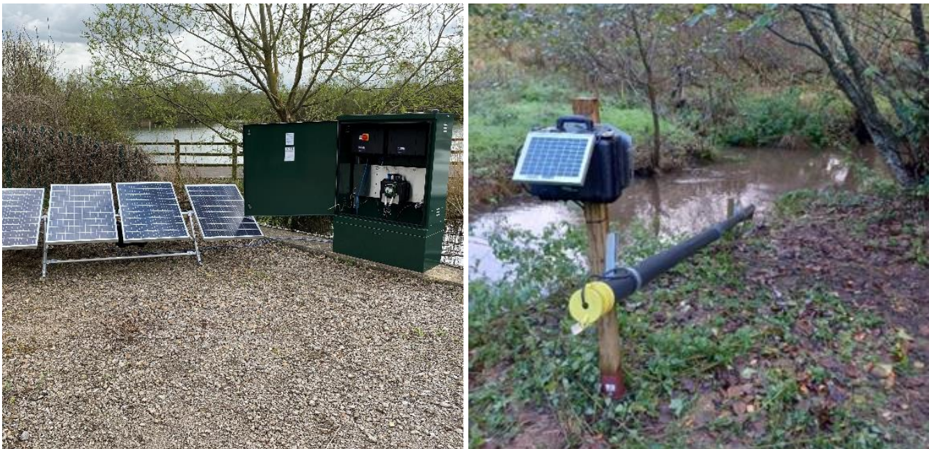
Figure 75 - Example of pumped kiosk installation (left) and in-river installation (right)
