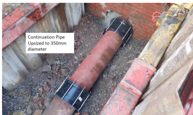
Figure 20 - Increasing capacity of the continuation pipe
