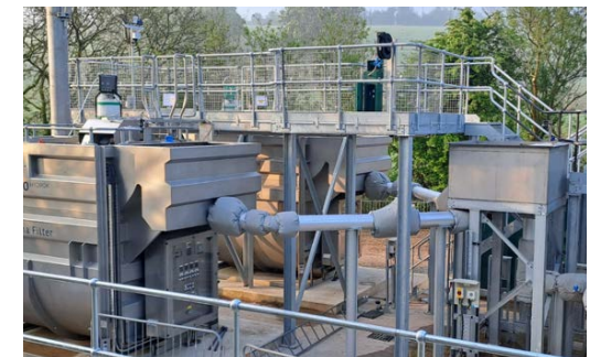
Pile cloth filter, that is a mechanical process for the separation of organic and inorganic solids from liquids.
