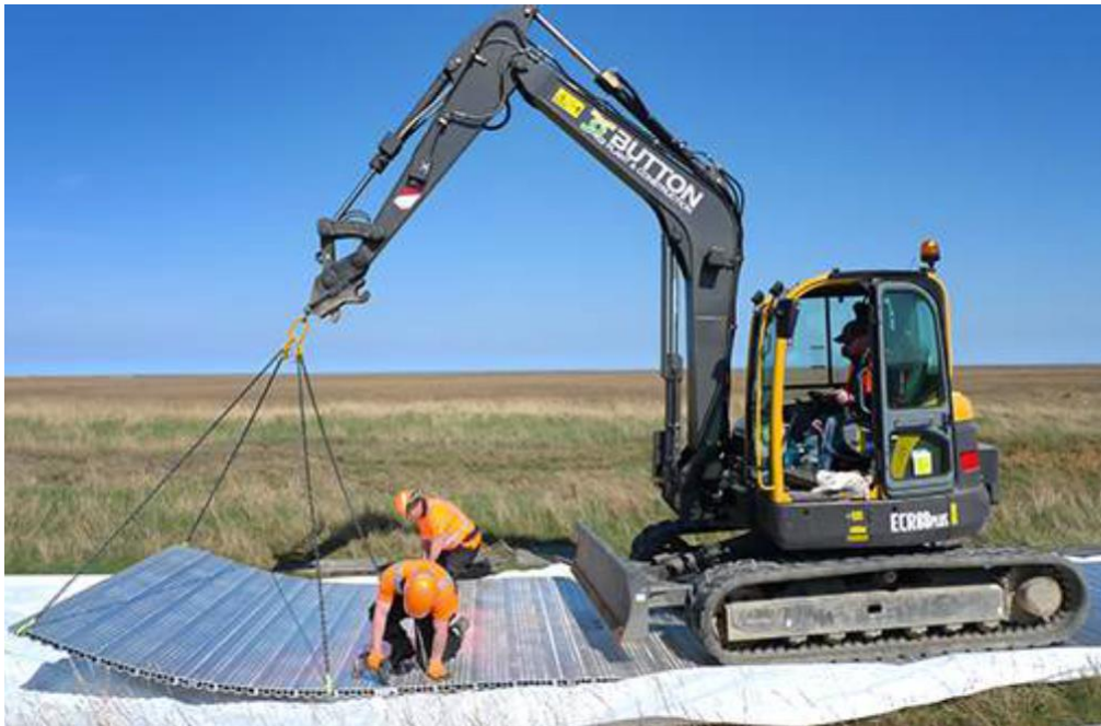
Figure 12 Example of Trackway temporary road across a SSSI
