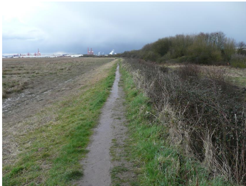
Figure 3 Picture showing scrub on landward side of the wall
