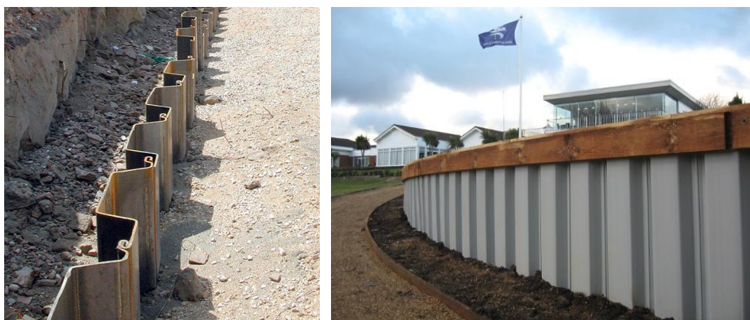
Figure 15. Steel and PVC interlocking trench sheeters
