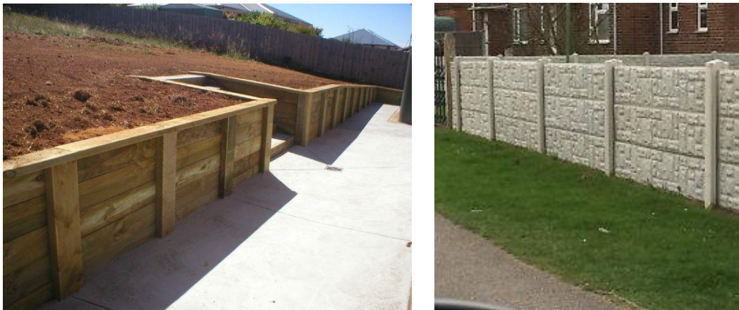
Figure 13. Wooden and Concrete Post and Plank Systems
