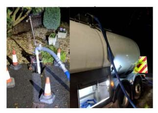
Tanker being used to supply over 50 properties in Taunton, via a hydrant, to allow a leak to be repaired without any one's water being turned off.
