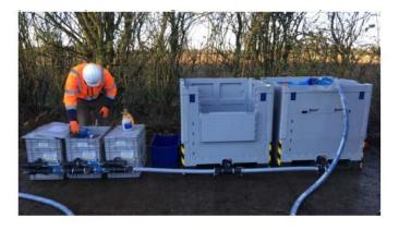
Temporary tanks with pumps to resupply an area can be delivered with a small van and positioned in places where a large tanker would be difficult to park.
