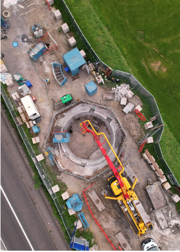
A new below-ground storm tank, capable of holding 125,000 litres of storm water, has been installed in the car park of Bath RFC's rugby ground at Lambridge.
