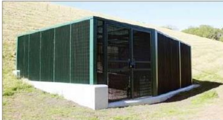
Figure 8-7: Typical physical protection barrier
